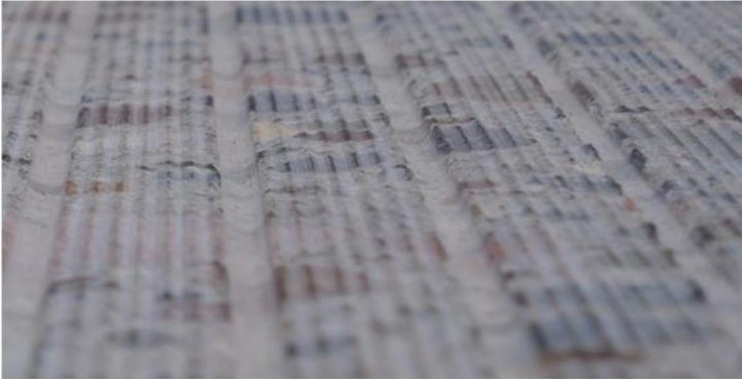
**Abbildung 17: Next generation Concrete Surface LITE (NGCS Lite) MnROAD Cell 37 [4]**
